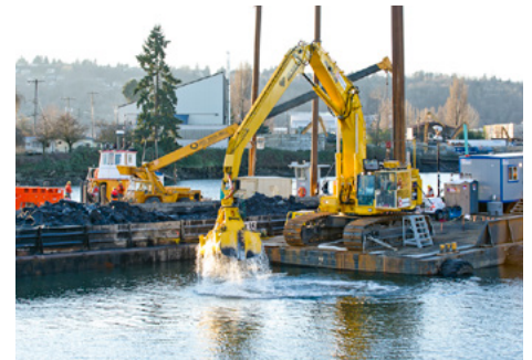
Boeing completed the first phase of removing contaminated sediment and replacing it with clean sand along a half-mile stretch of the Lower Duwamish Waterway. (Boeing photo)
