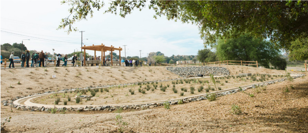
A biofilter storm water treatment system uses natural processes to capture pollutants before releasing cleaner water back into the watershed at the Santa Susana remediation site. (Boeing photo)
