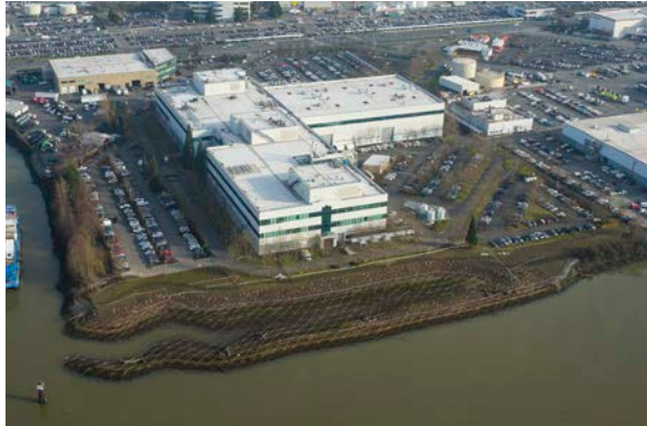
Boeing restored nearly one mile (1.6 kilometers) of former industrial shoreline, creating habitat to support fish and wildlife in the Lower Duwamish Waterway. (Boeing photo)
